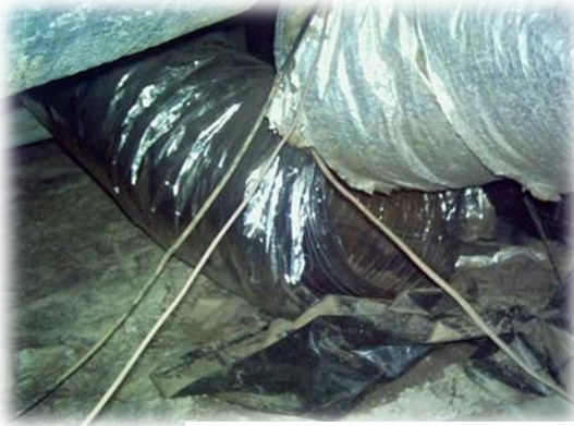
Disconnected Duct
