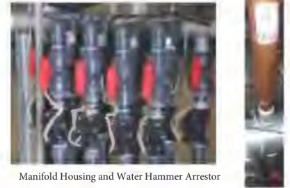
Manifold Housing and Water Hammer Arrester
